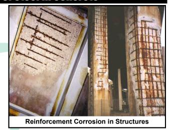
reaction reduces the alkalinity of the concrete that protects the steel. When the pH at the level of the reinforcing steel falls below 9, corrosion begins. Chloride-induced corrosion is more common than that resulting from carbonation.
