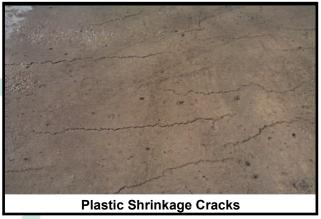
Conditions that cause high evaporation rates from the concrete surface, and thereby increase the possibility of plastic shrinkage cracking, include:
