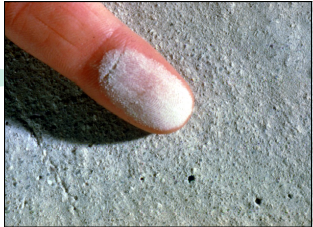
Dusting concrete surface
