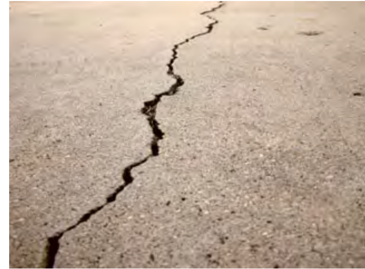
Structural Cracking (Widened)
