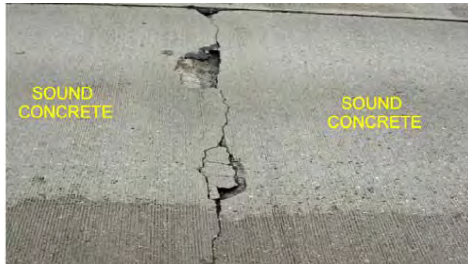
Structural Cracking (Spalled)
