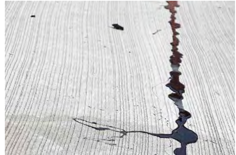
Crack Sealing – An Example of What NOT To Do!
