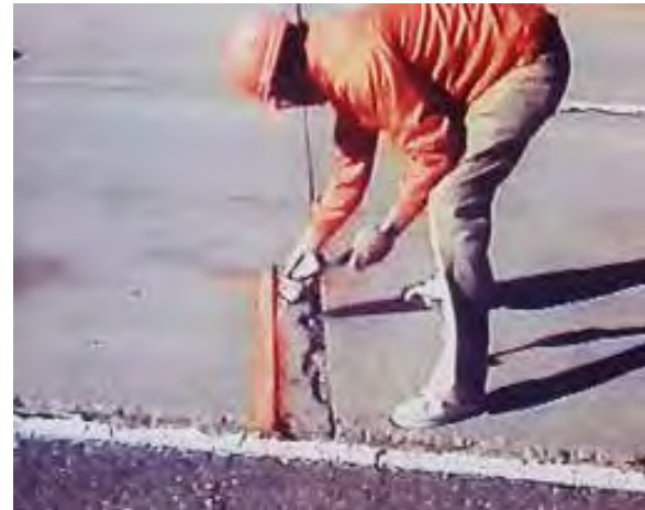
Marking area for removal
