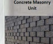
Concrete Masonry Units are stackable hollow concrete blocks that are manufacture in many different heights, lengths and angles that can give the end product a custom look.
