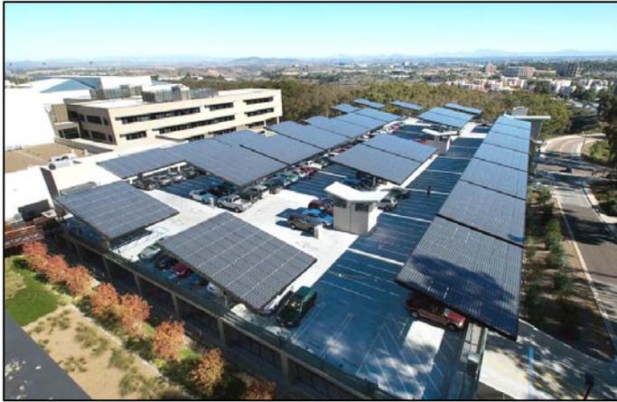
**Figure 3. Hopkins Parking Structure at the UC San Diego Campus Illustrating Photovoltaic Cells for Parking Lot Canopies and High Albedo Concrete in the Driving Lanes.**
