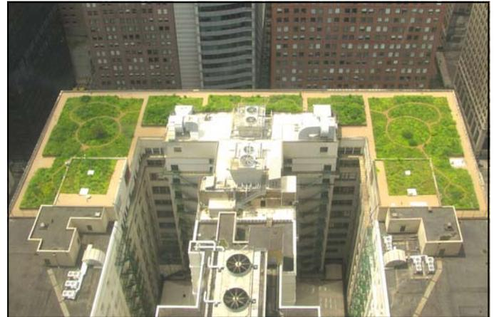
**Figure 4. Green roofs, such as Chicago City Hall's, help reduce urban heat islands through evapotranspiration and reducing heat gains and losses through the roof.**
