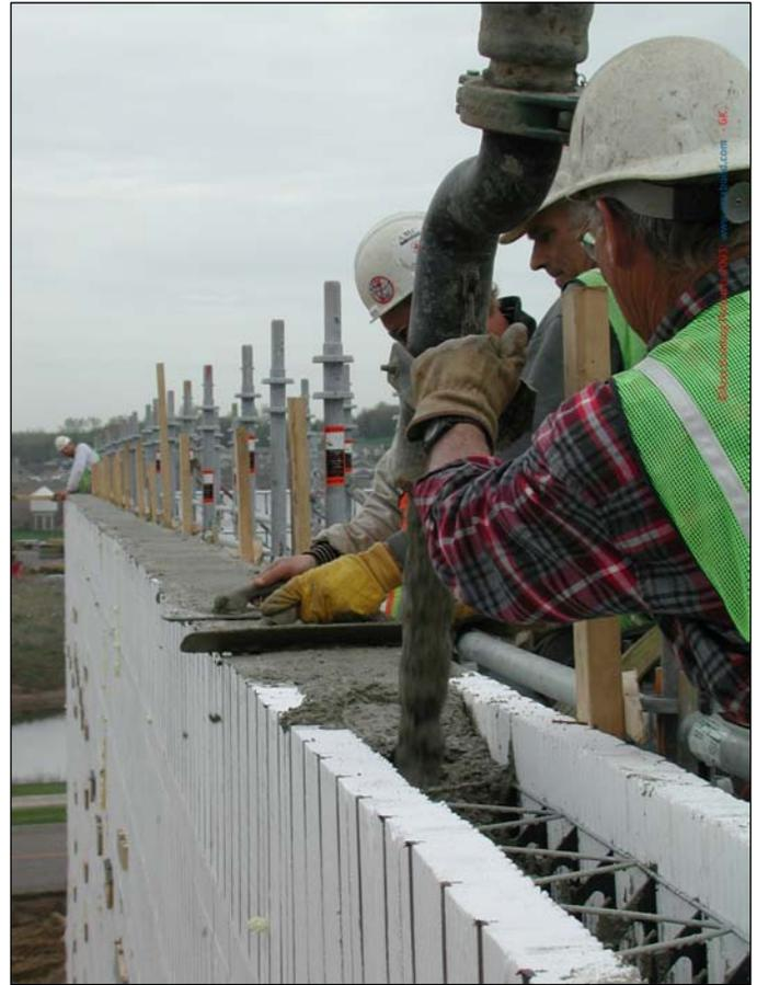
*Figure 4. High performance concrete building systems such as insulating concrete forms, tilt-up concrete and concrete frame construction help a building meet the requirements of LEED 2009 NC energy performance requirements.*
