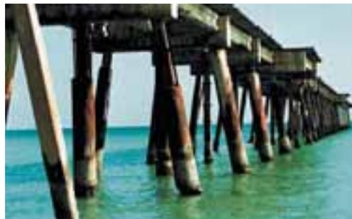
Figure 4. Corrosion of steel rebar due to chloride ingress
