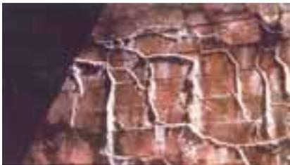
Figure 6. Cracking of a concrete bridge substructure due to ASR
