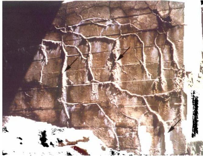
**Figure 5. Cracking of a concrete bridge substructure due to ASR**
