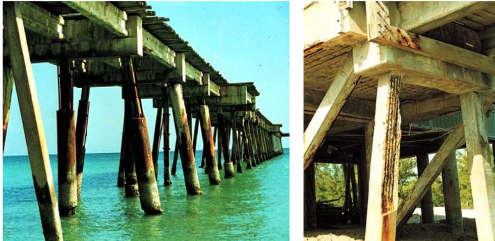
**Figure 4. Corrosion of Steel Rebar Due to Chloride Ingress**
