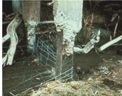
*Figure 2: Example of deterioration of concrete due to exposure to sulfates.*
