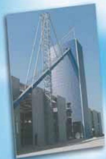
Only SIMEM offers prefabricated plants of both horizontal and vertical arrangements. Our Beton Tower® prefabricated high output vertical plant can store 1400 tons of aggregate storage overhead, and full enclosure, yet install in a few weeks time, fully wired and plumbed!
