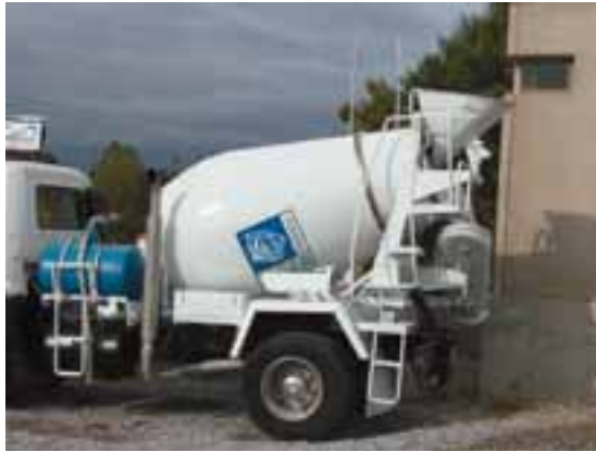
Ready Mixed Concrete Truck used to Prepare the Concrete
