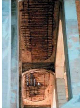
Examples of corrosion of reinforcing steel in concrete structures.
