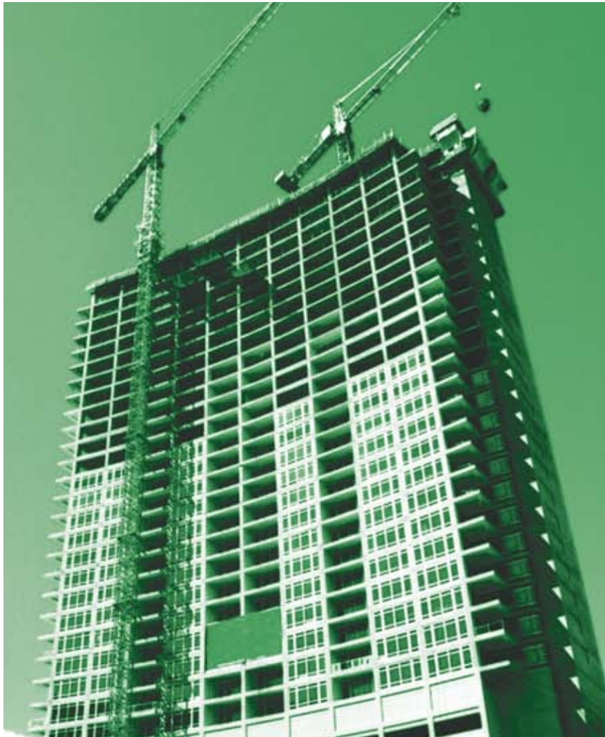
Figure 4: Building under construction.
