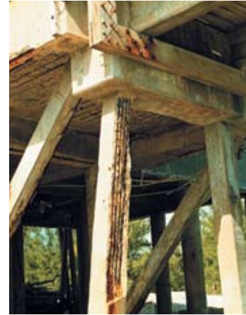
Examples of corrosion of reinforcing steel in concrete structures.
