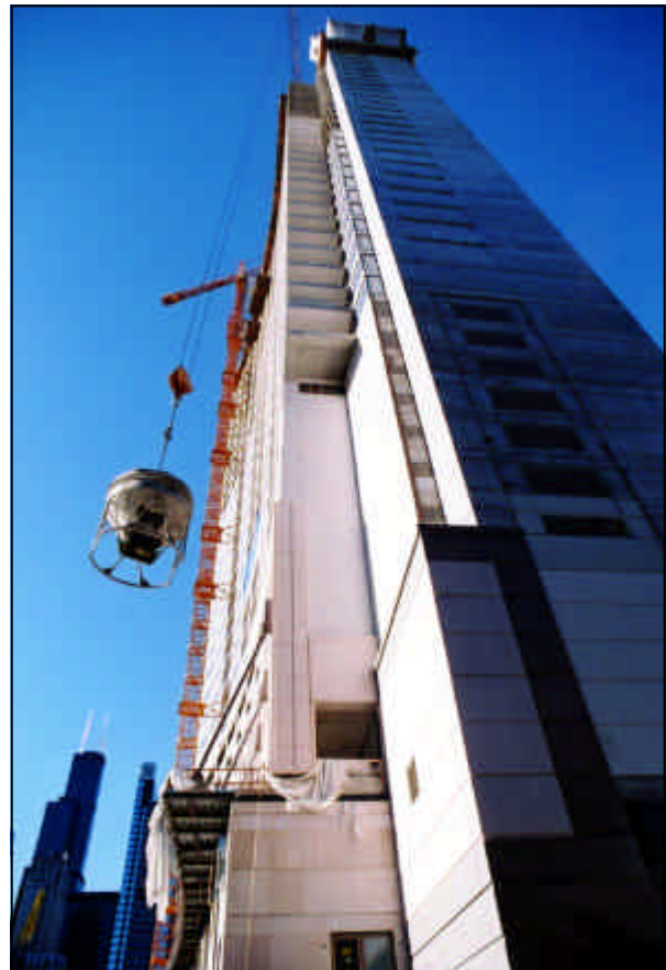
Figure 1. Performance-based specifications foster innovation and acceptance of new technology such as high-strength concrete and self-consolidating concrete for high-rise construction.
